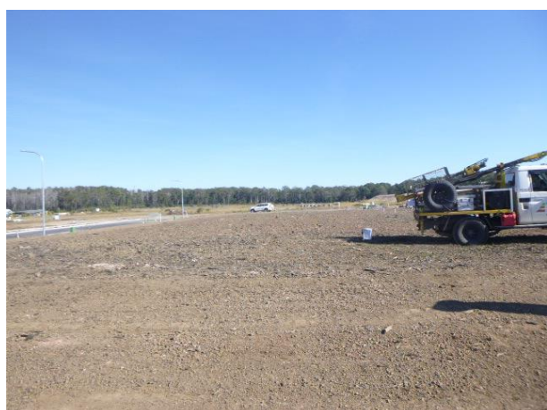
View west from Lot 44, showing regraded site following fill placement.
