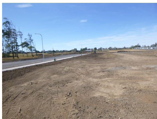
View east from Lot 60 showing flat to gentle slopes towards the south east.
