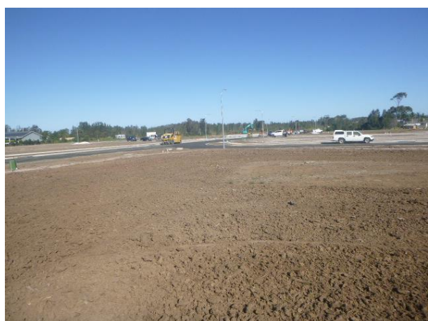
View south east from Lot 19, showing regraded site following fill placement
